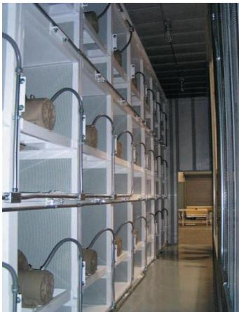
A FanWall air handling unit consists of an array of smaller fans moving air through a system. The FanWall AHU has been proven to reduce AHU energy usage, vibration, and reduce footprint of equipment. In a conversation with the engineer, it was mentioned that Penn State was unwilling to risk using FanWall AHU because of their inexperience with the equipment and the potential for extra maintenance needed for each fan, despite reliability claims from HUNTAIR, the manufacturer of FanWall.
